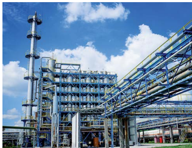
Column; \varnothing 1.4 \text{ m} ; H = 42 \text{ m} ; Weight \approx 54 \text{ t}
